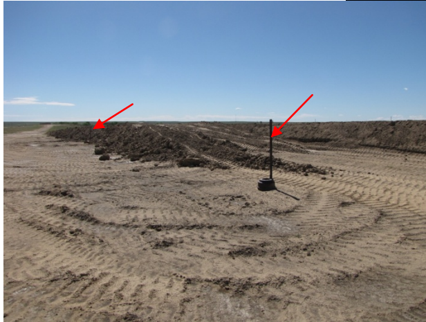
Photo 1 – Soil Depth Markers for Coverfill
