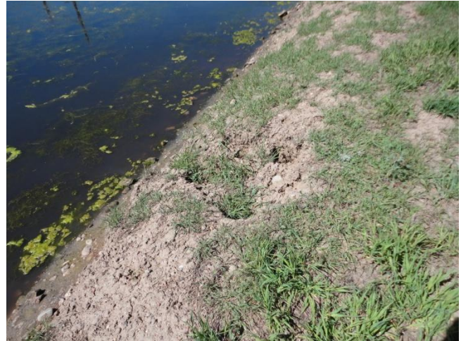
Slumping along Pond 5-P7 embankment.
