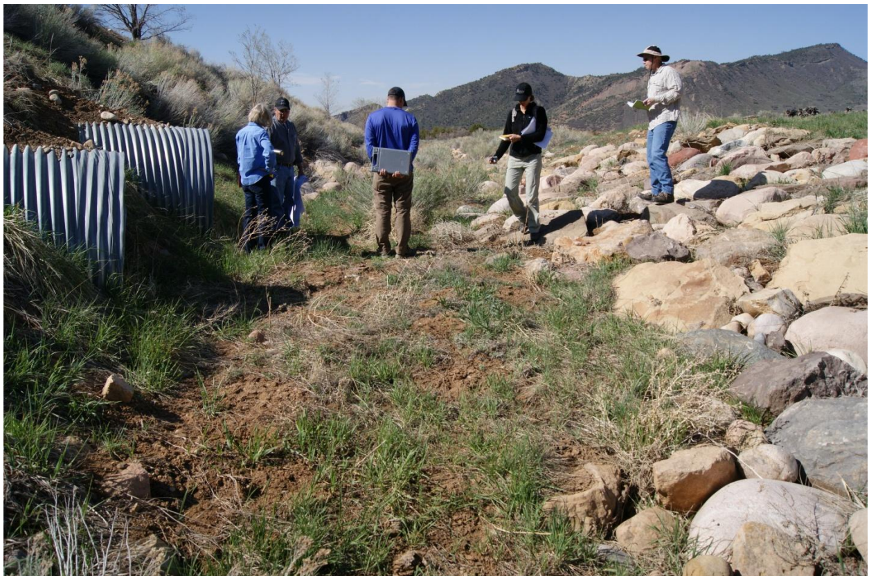
Permanent diversion channel at outlet of twin 66" CMPs
