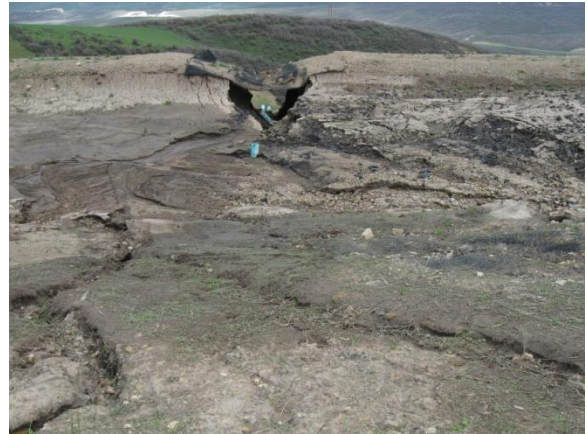
Lower surge tank in YPM-13 drainage. Damaged and need repair.
