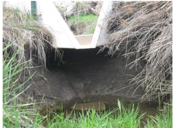
Small drainage undercutting the flume at Pond 014. Need repair.
