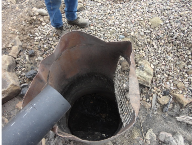
Photo 37: Drop inlet 2 to be cleaned
