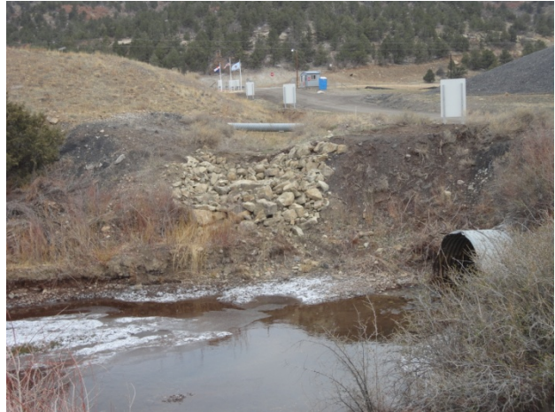
Photo 28: Armoring to replace gabion at D10 outlet
