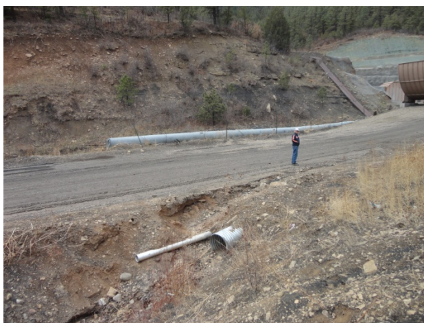
Photo 34: C48 in the background, unidentified culvert conveying disturbed area runoff in front
