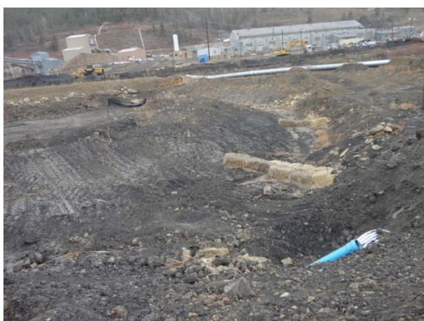
Photo 24: Open channel replacing C26
