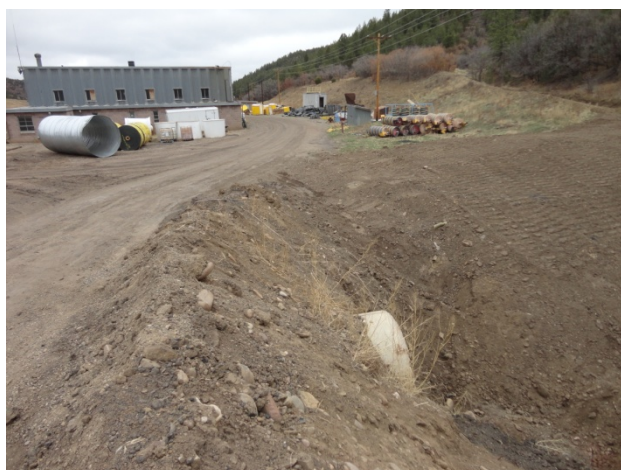
Photo 11: Berm needed to protect C2 inlet
