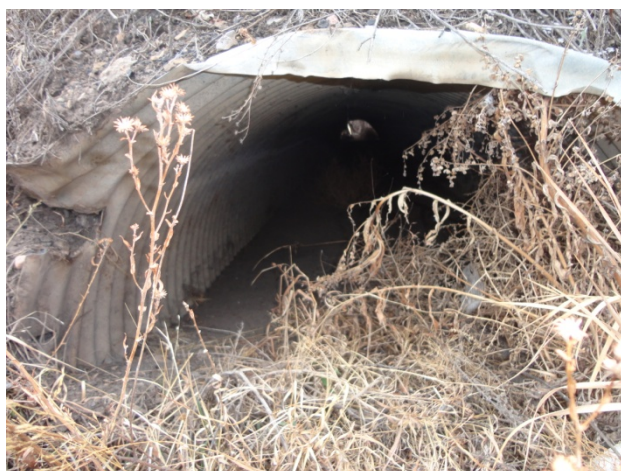
Photo 33: "Railroad culvert", needs to be cleaned
