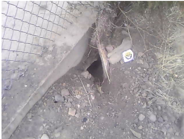
Photo 41: Slumping at airshaft pad to be filled
