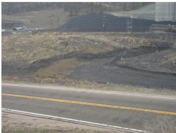
Photo 22: Berm at edge of disturbed area north of containment 3
