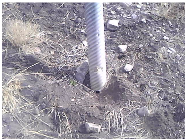
Photo 3: Primary spillway riser, pond 9/9b
