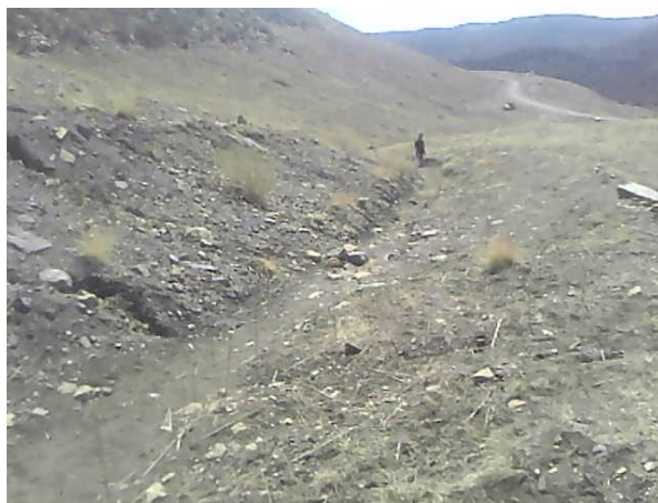
Photo 8: Ditch near fill 7 needing flow control
