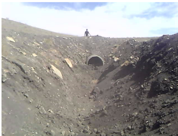
Photo 7: Concrete culvert
