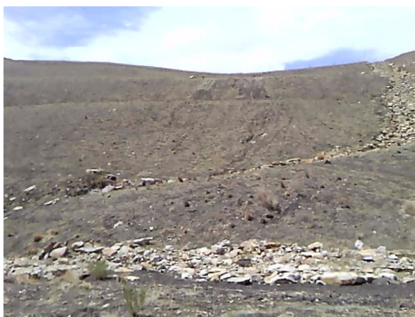
Photo 9: Gully and rills on fill 9 needing repair
