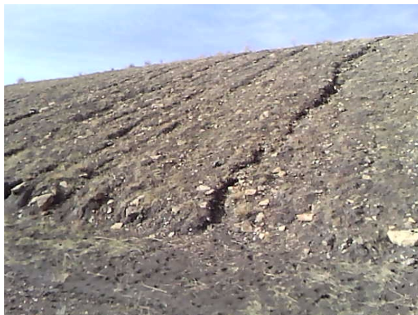
Photo 2: Vegetated rills on fill 9 to be monitored
