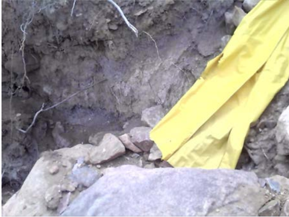
Photo 11: bottom of sock where water is cutting into South bank below culvert 1S Monarch fan road.
