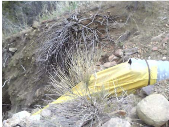
Photo 8: junction of Culvert 1S on Monarch fan road With "sock"
