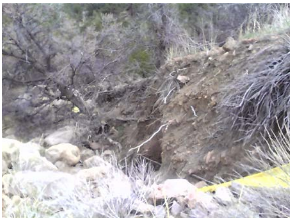
Photo 9: bank cutting on south side of Culvert 1S outfall
