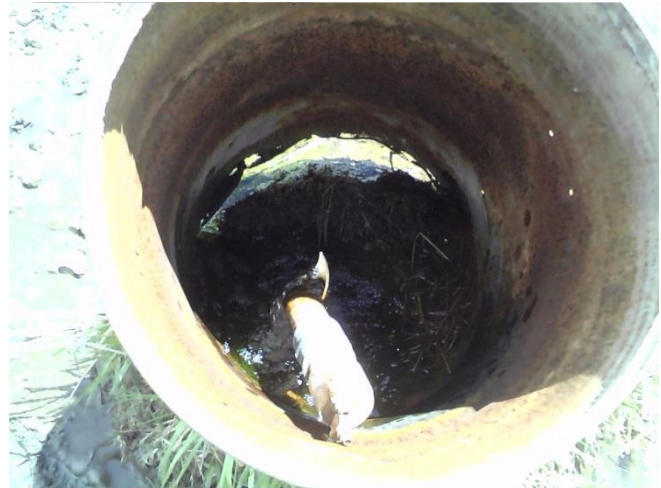
Damaged Well Head
