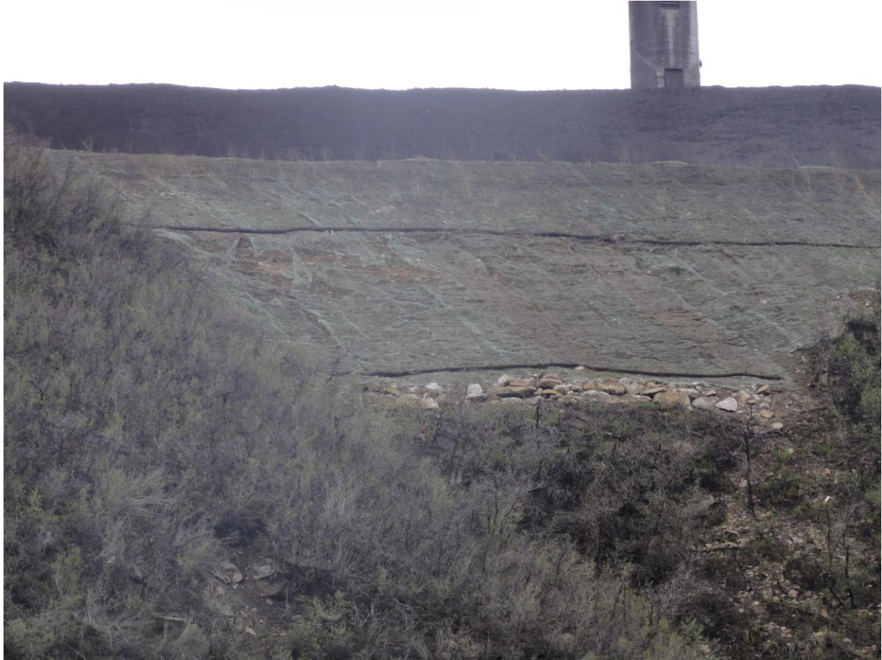
ST-02 repaired slide area
