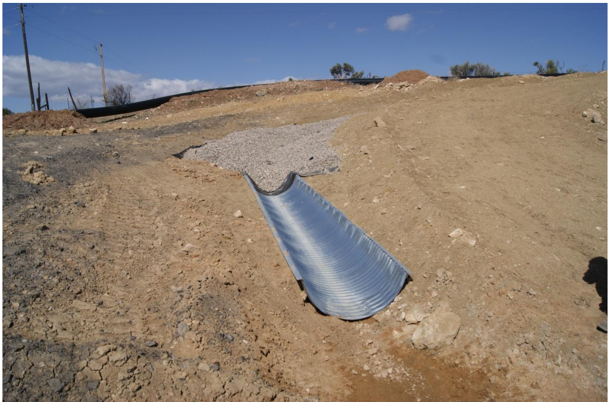
Photo 4 – 36-inch half-pipe run-down – SW corner of Pond NHN-001
