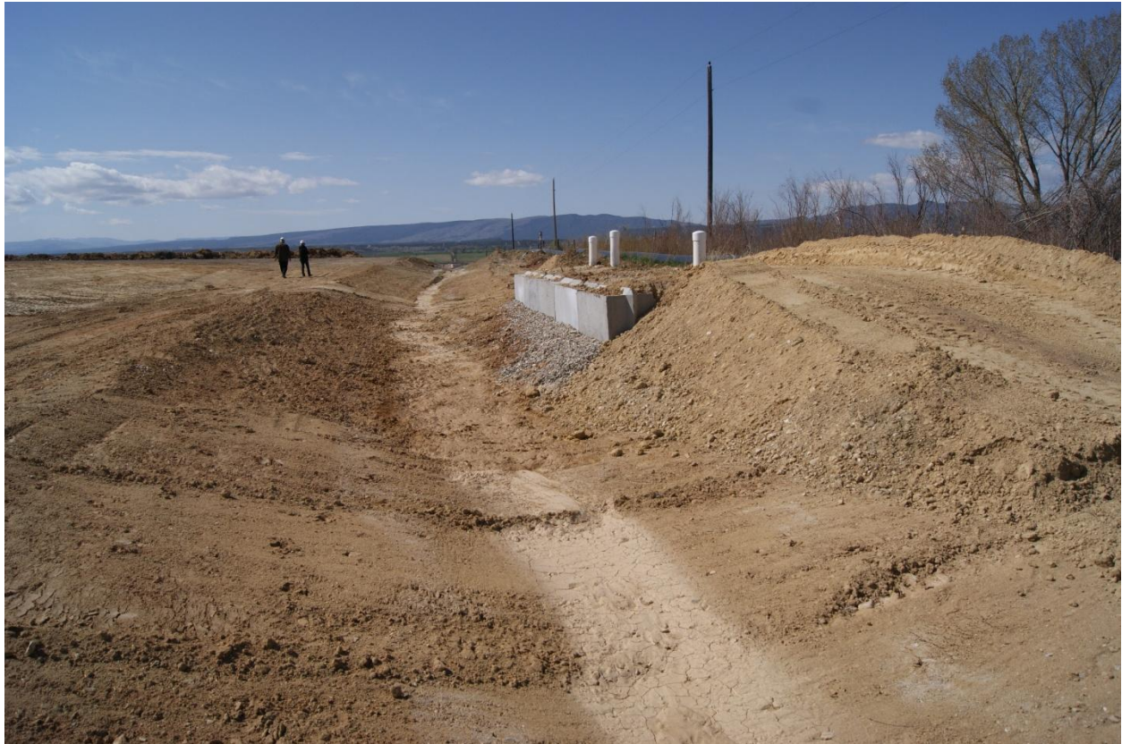
Photo 5 – Monitoring wells, and flatter portion of Ditch NHN-001-West, looking south
