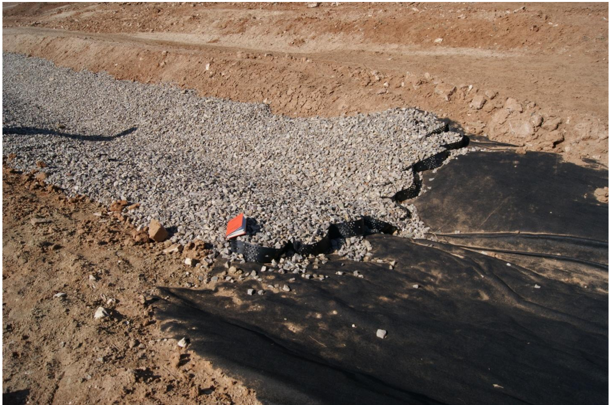
Photo 3 – V-Bottom Ditch Lining
