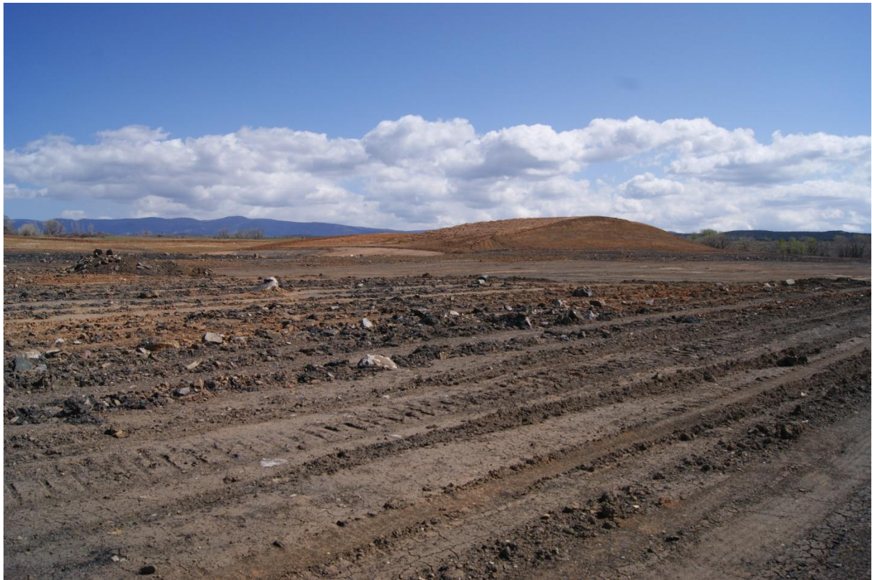
Photo 1 – Surface roughening, looking NE toward REC stockpile
