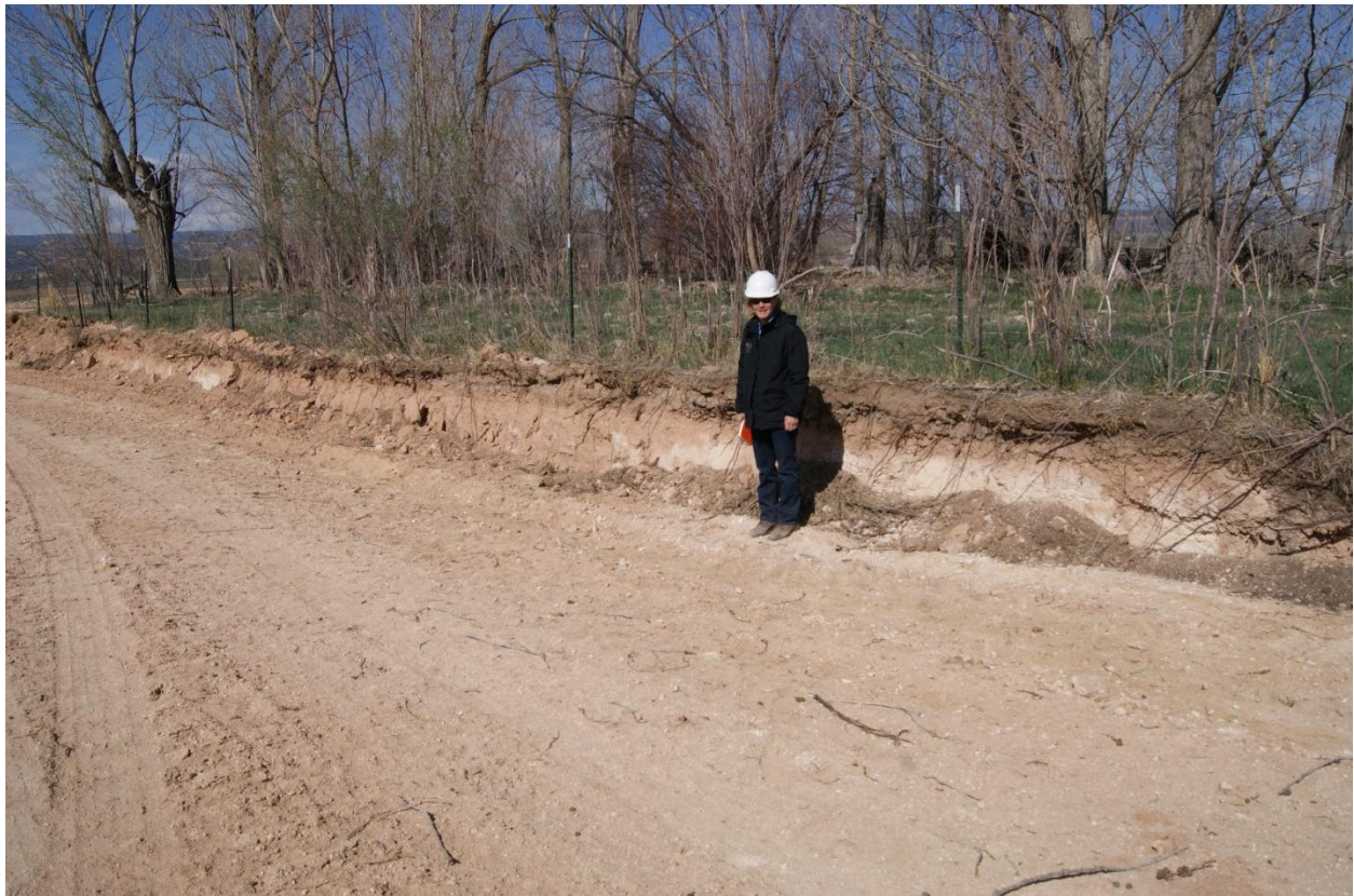
Photo 8 – Topsoil depth – northern limit of area that has been stripped
