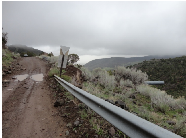
Standing water at location of blocked West Mine culvert
