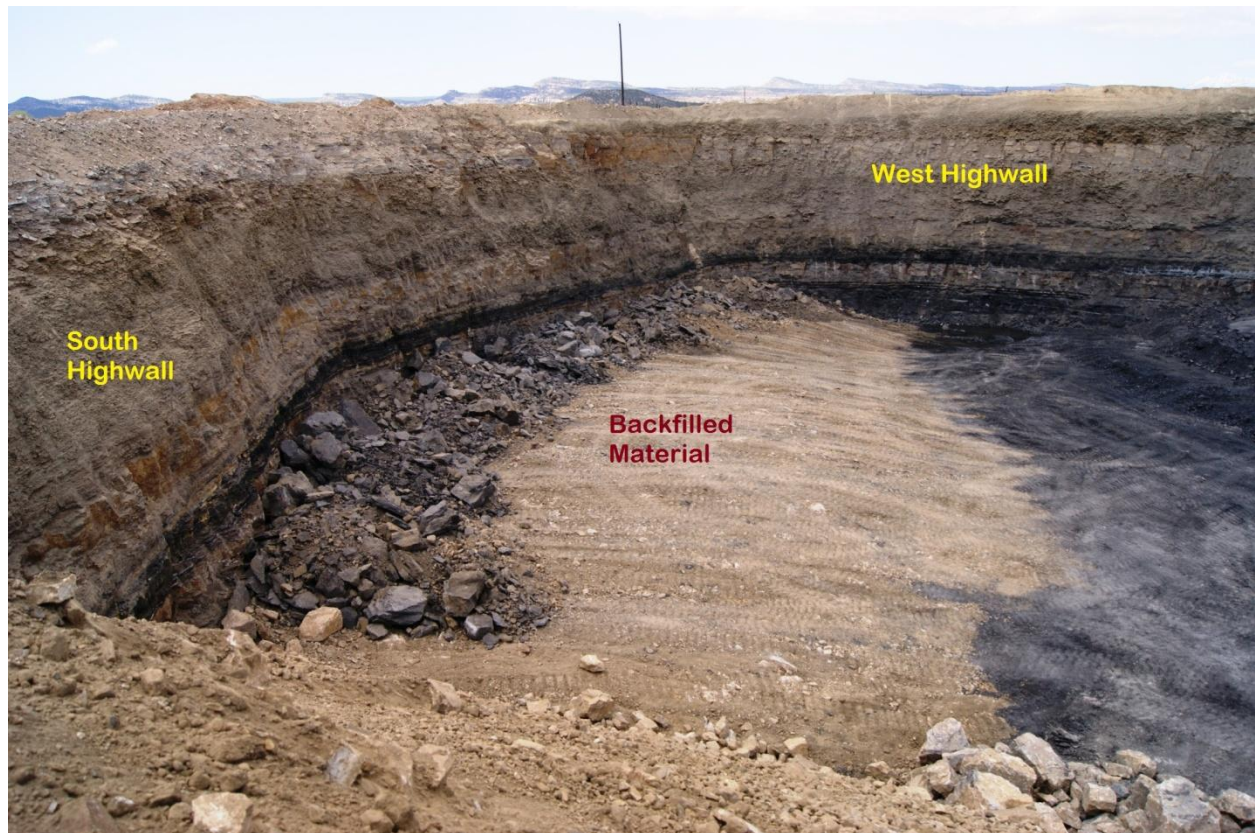
Photo 1 – Early stages of backfilling final highwall on WFC property
