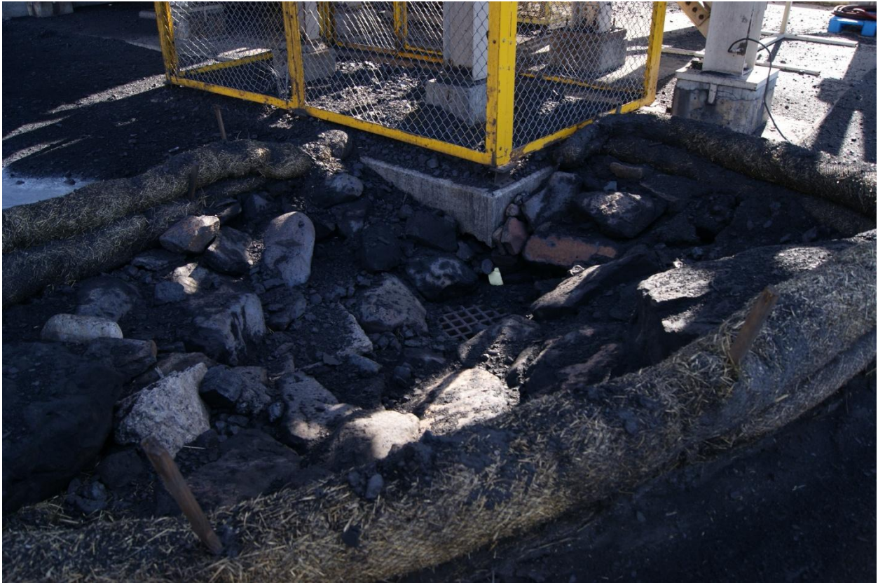
Photo 3 – Grated drop inlet at foot of screening tower
