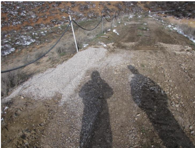
Backfilled sink hole in Pond DP-1 embankment.
