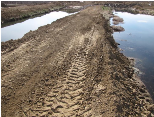
B-Seam dewatering pond embankment repair.
