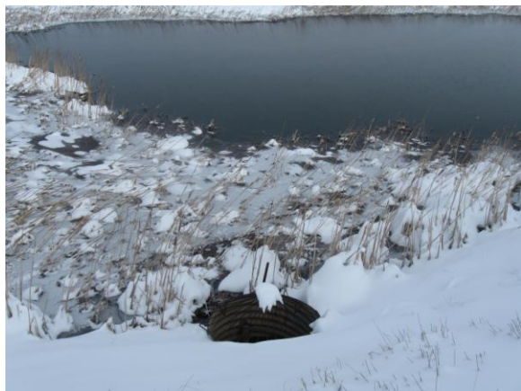
Impoundment H, primary spillway culvert.
