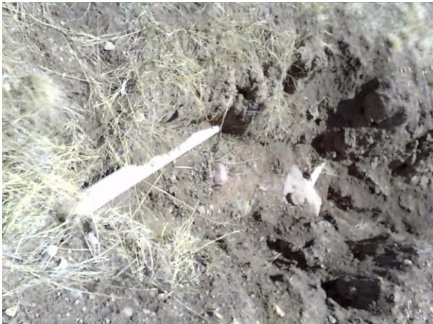
Photo 9: Exposed PVC pipe in gully
