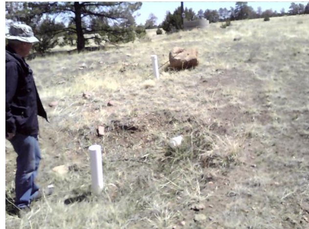
Photo 10: Protruding PVC near well 119459
