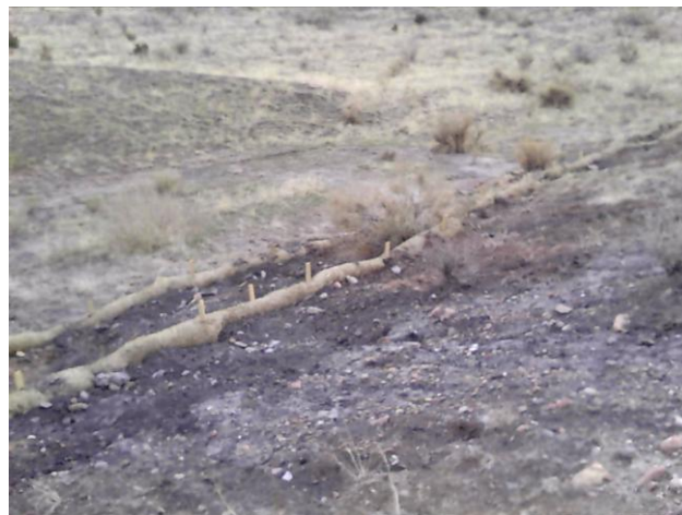
Photo 24: wattles placed on slope
