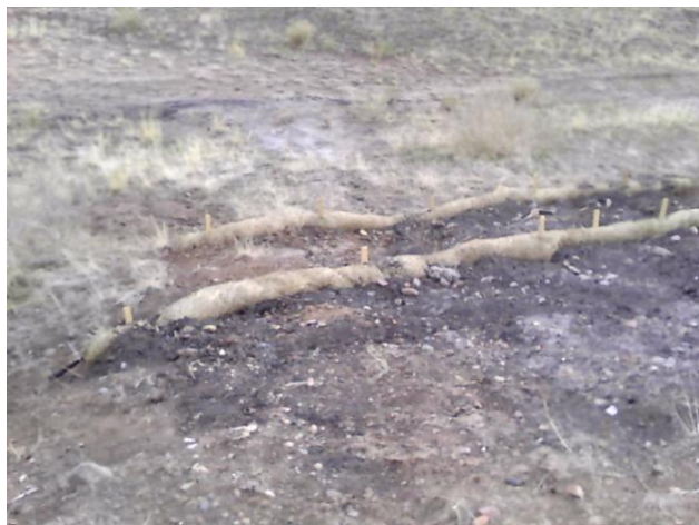
Photo 23: wattles placed on slope
