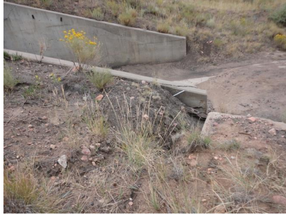
Photo 6: NE corner of truck tunnel needs erosion control measure.
