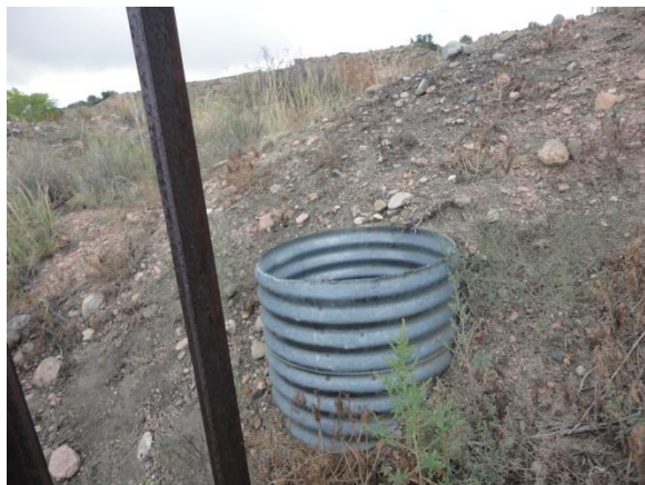
Photo 11: slope sloughing into pond L1 riser
