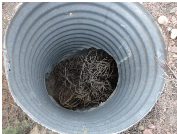
Photo 12: material sloughing into Pond L1 riser
