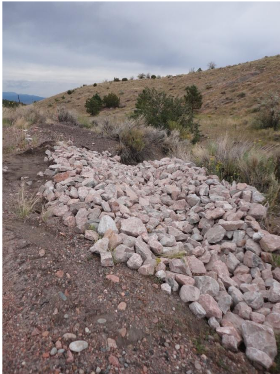
Photo 3: rock armoring at Access rd. drainage
