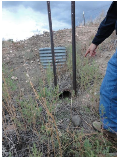
Photo 10: gated valve missing from pond L1 riser @ loadout
