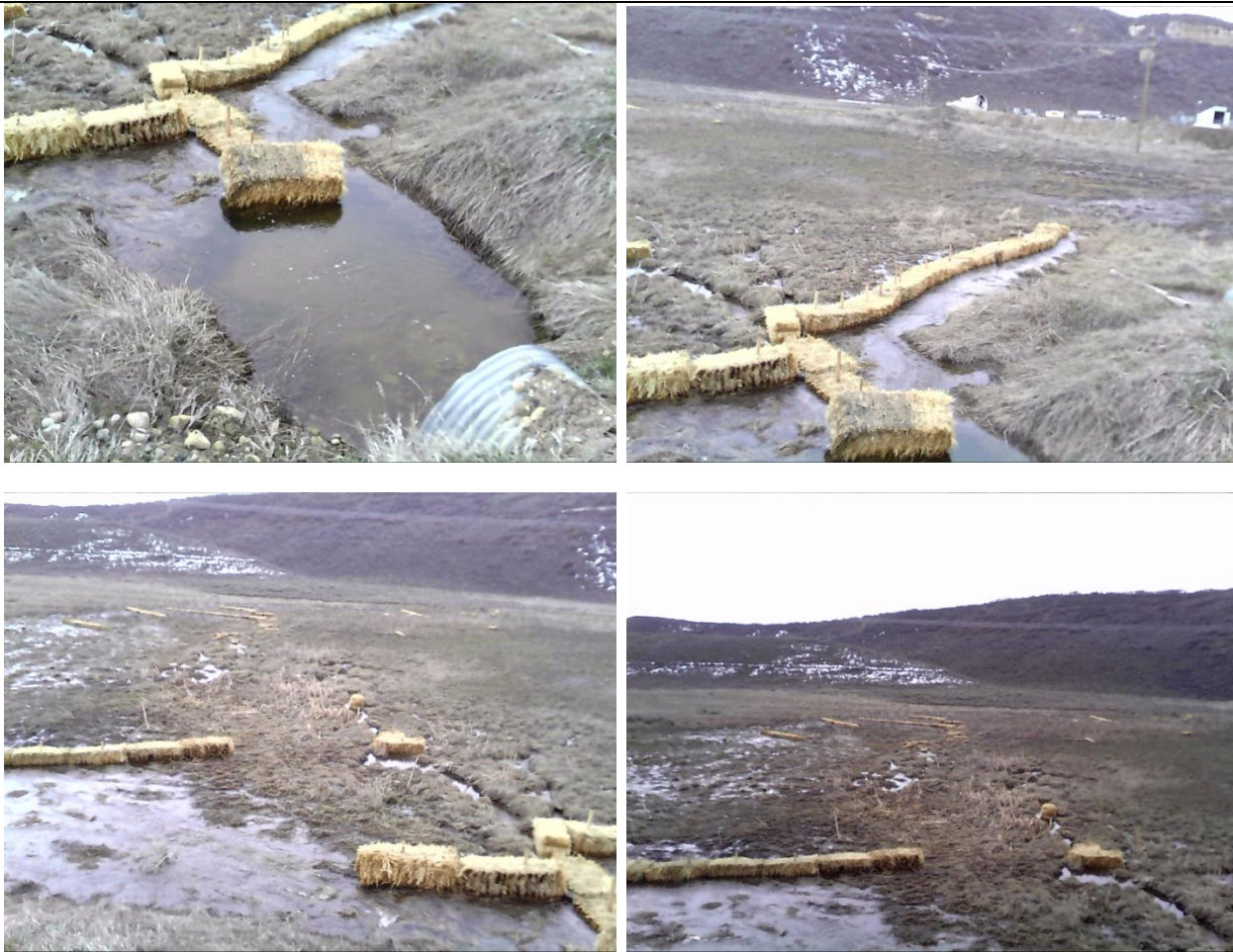
Installed Straw Bales
