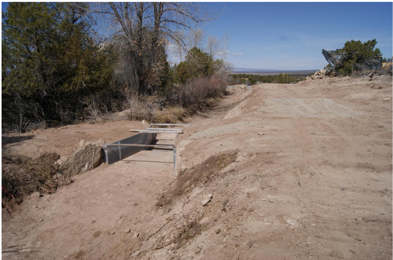
Photo 2 – Second Park Lateral ditch and Parshall flume, looking downstream toward box
