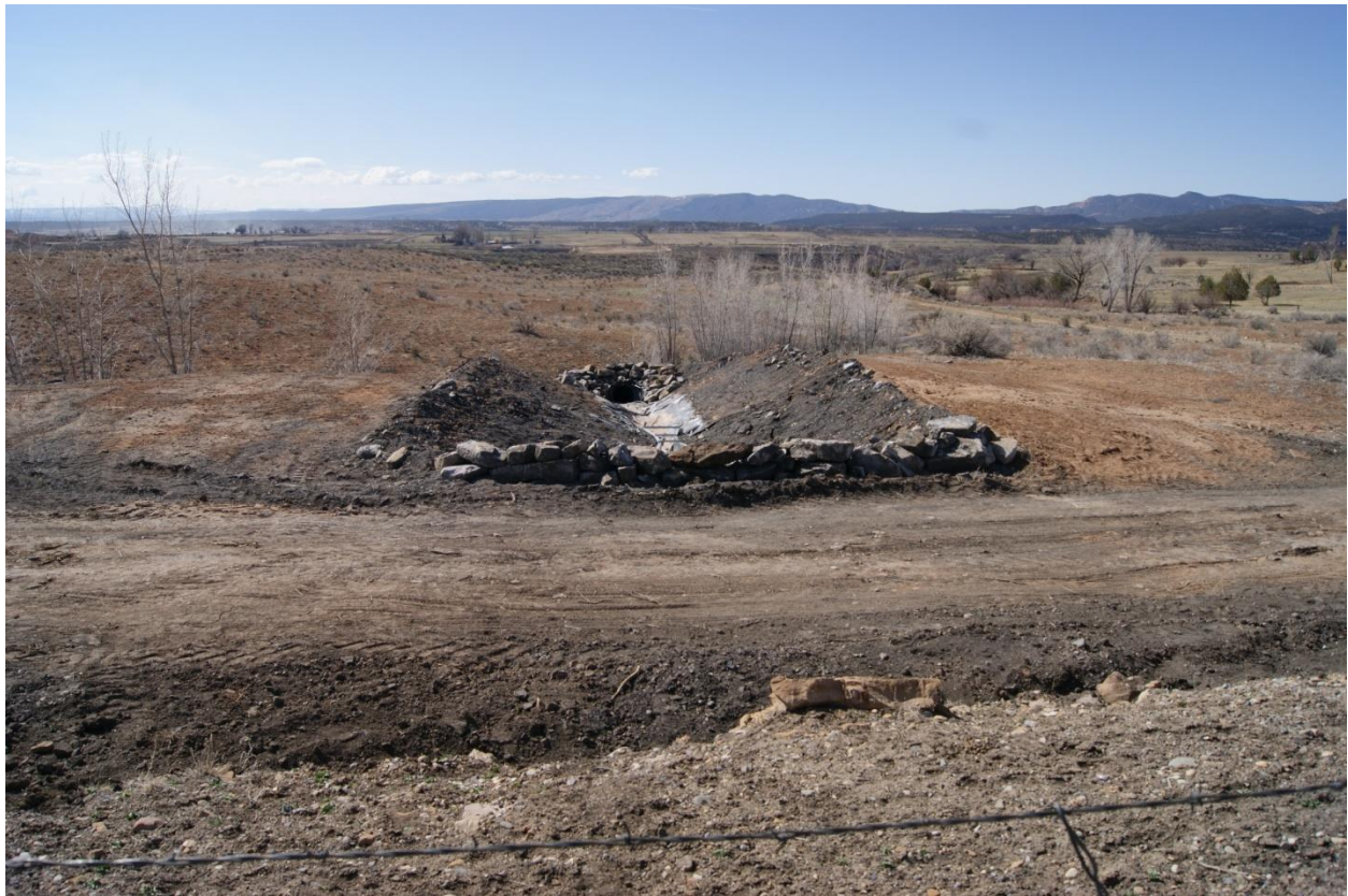
Photo 3 – Pond NHN-001 outflow ditch, looking S from AA Road
