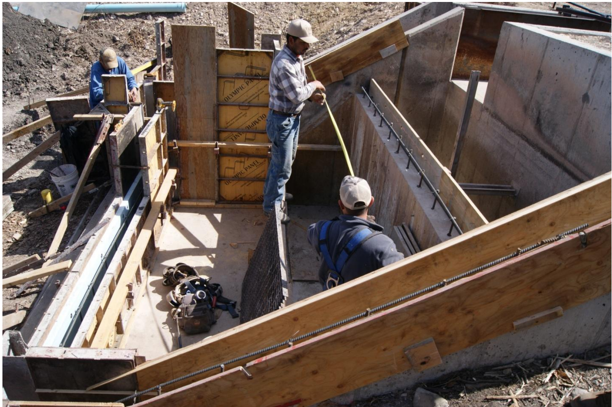
Photo 1 – Construction crew at Second Park Lateral ditch division box
