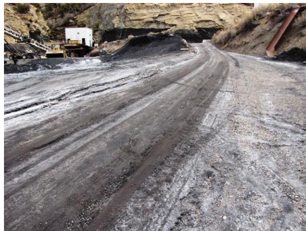
Photo No. 3 – Minor rills at upper end of haul road & stockpile areas.
