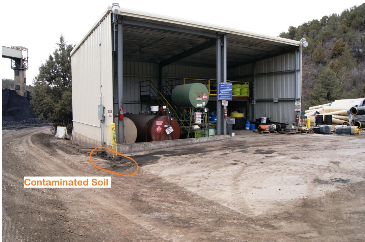
Photo 4 – Petroleum storage shed, contaminated soil
