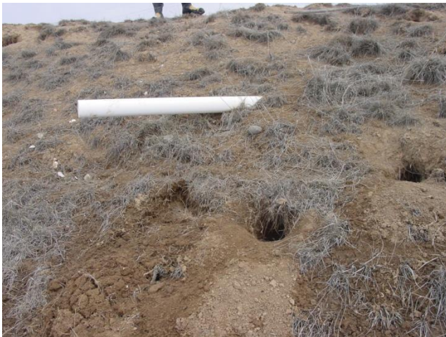
Rodent holes in Pond 9-P8's embankment.
