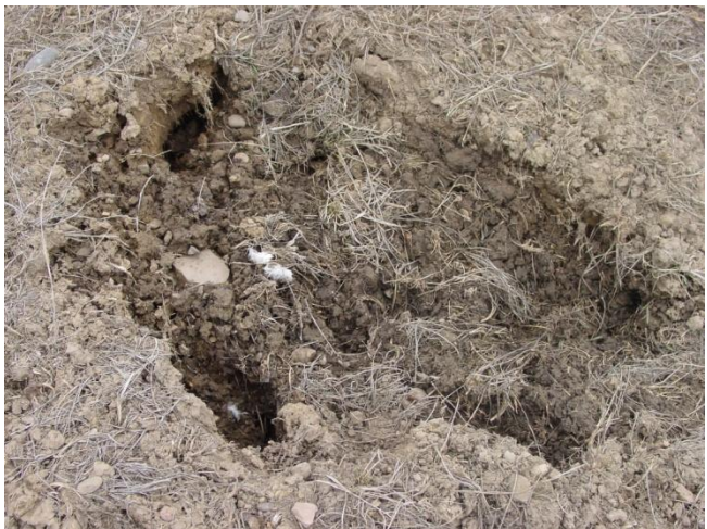
Sink hole in Pond 5-P7 embankment.
