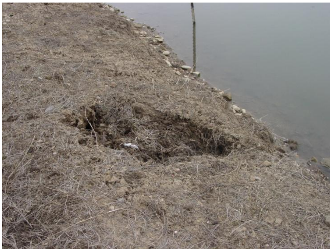
Sink hole in Pond 5-P7 embankment.
