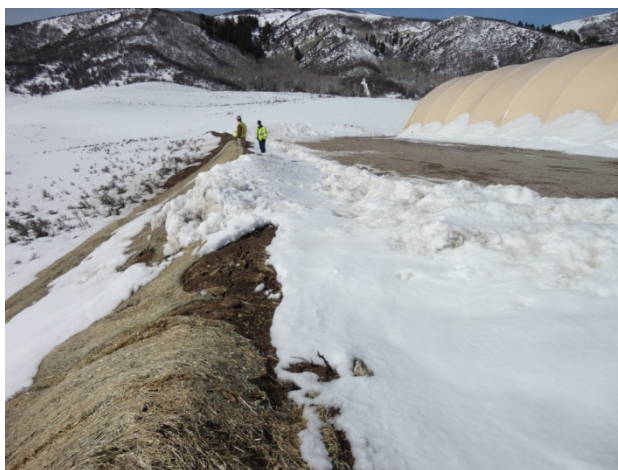
Photo 4: Slump in berm at the 16-Left Utility borehole pad SAE
