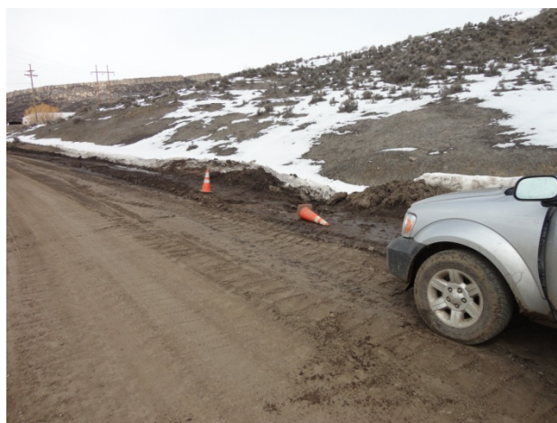
Photo 10: Breach in roadside ditch
