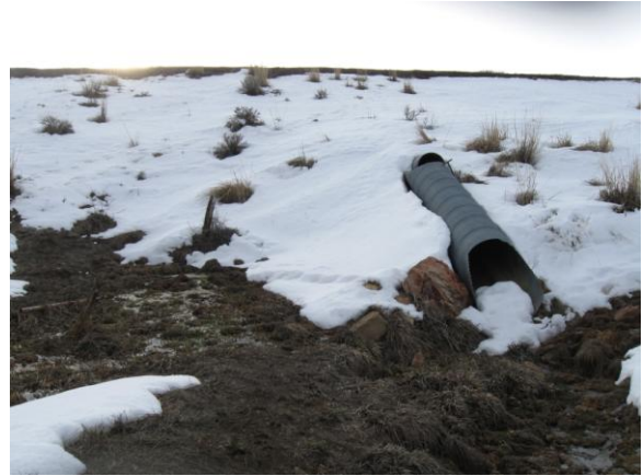
Pond 005 primary spillway at the base of the embankment.
