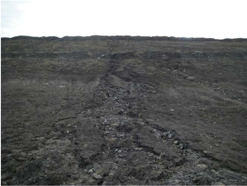
Blowout of contour ditch above confluence of East Taylor Ditch and Taylor Tributary Ditch
