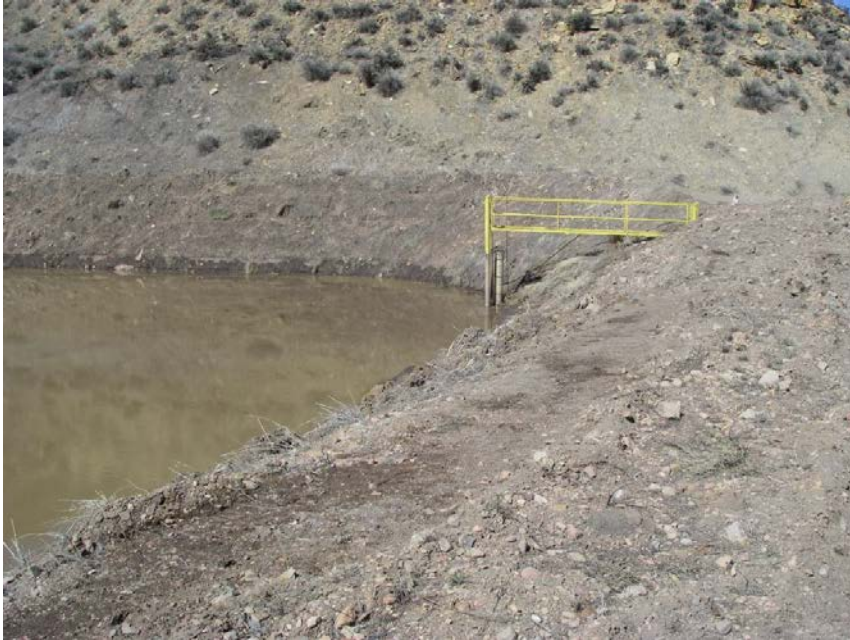
Prospect Pond embankment and primary spillway
