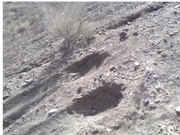
Photo 12: tire "divots" dug into pond L1 slope
