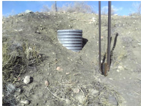
Photo 10: Pond L1 repaired primary riser & sealed gate.
