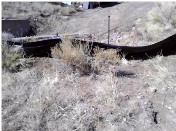
Photo 6: Silt fence well anchored at truck tunnel
