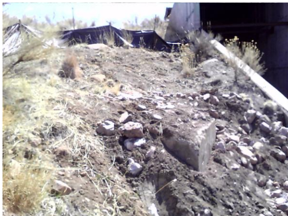
Photo 5: repair to rilling by truck tunnel
