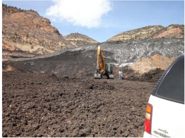
End dumped gob being moved, spread, and compacted
