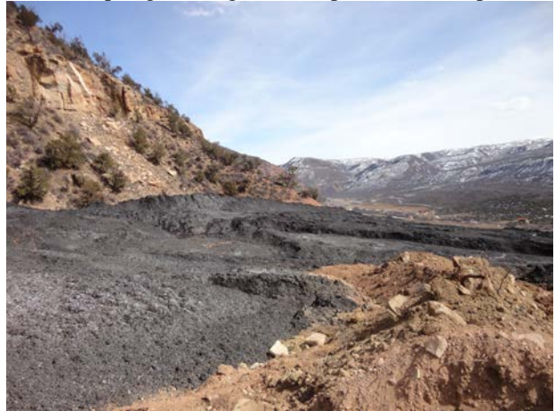
End dumped gob being moved, spread, and compacted
