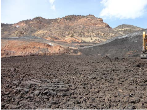
Gob Pile #2 – gob placed on former cover mat'l footprint
