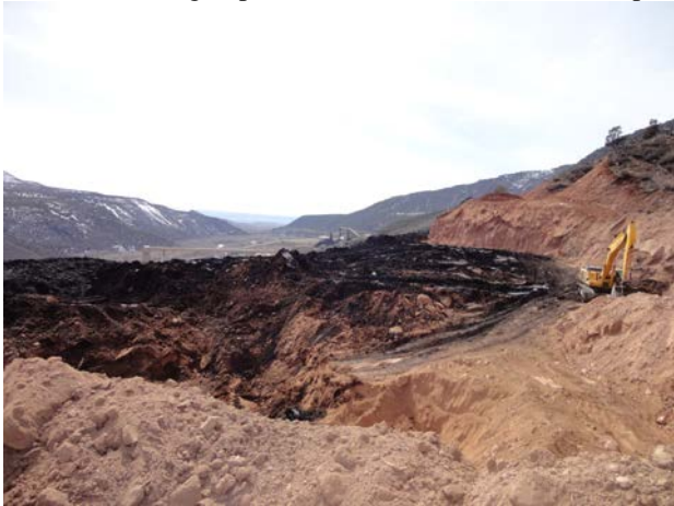
Gob Pile #2 – gob placed on former cover mat'l footprint
