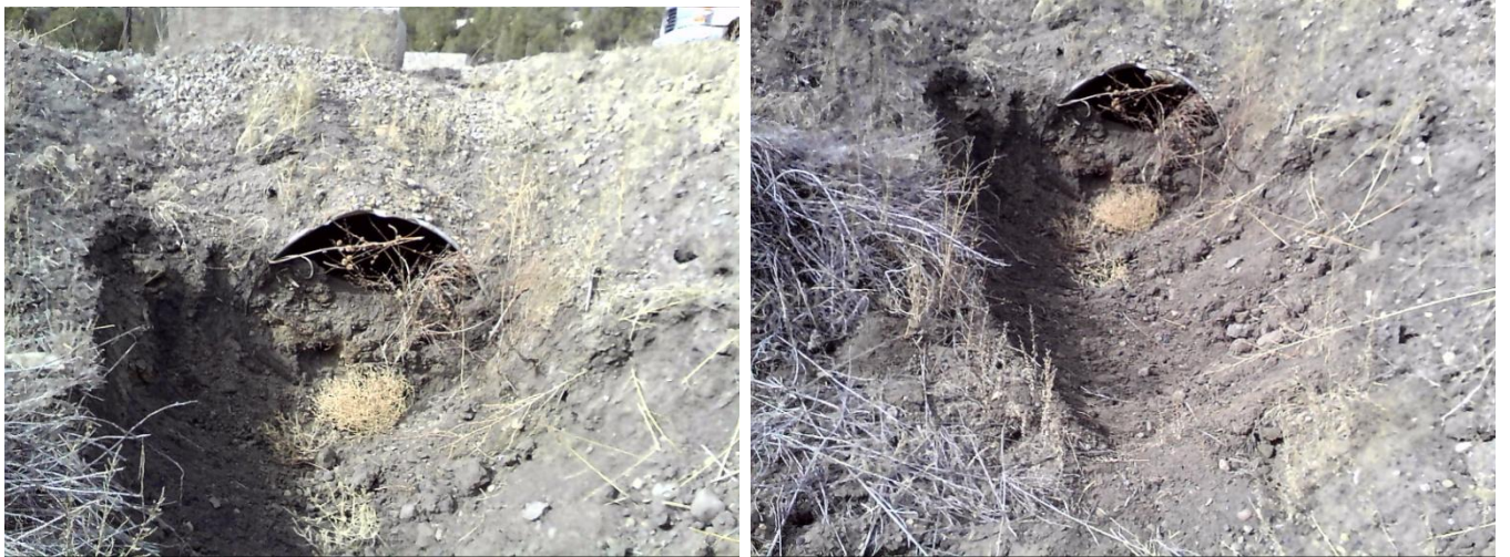
Culvert C-6 Inlet Clean-out and Sediment in Culvert
