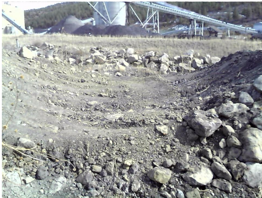
Area of Culvert C-26 Removal and Channel Establish
