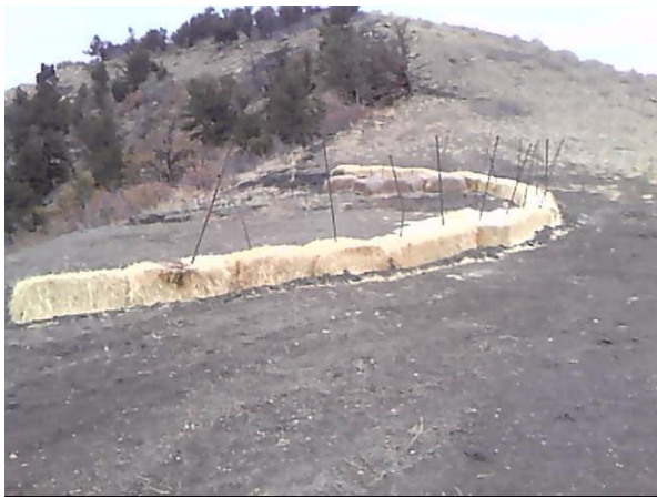
Hay bales above natural drainage to Pond 5.
