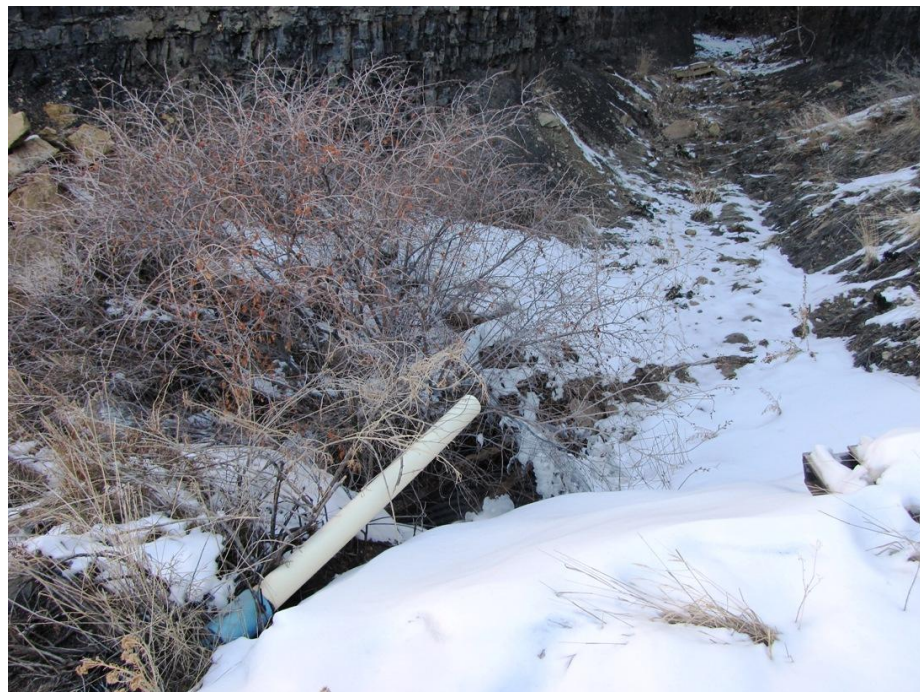
Mine Water Discharge Pipe
