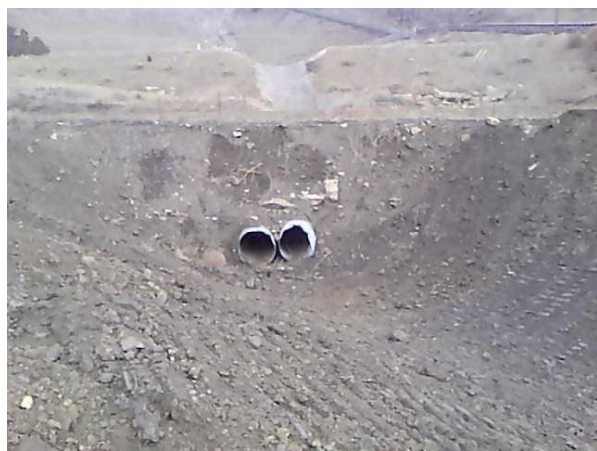
Reestablished drainage ditch east of Topsoil Pile SAE.
