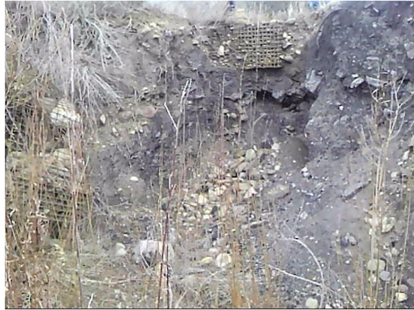
Erosion and cutting around gabions.
