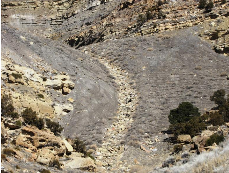
Photo No. 1 - Mine #1 outslope and drainage channel.
