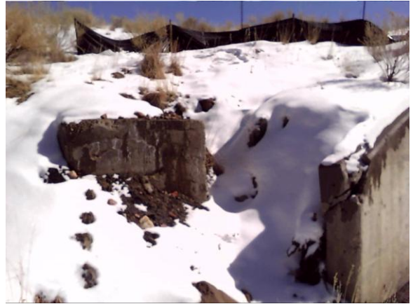
Photo 2: Silt fence at truck tunnel rill repair. Still need seeding for stabilization.
