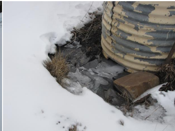
Photo 4 – Water Backed-Up at Outfall 001A
