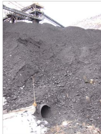
Photo 6 – Culvert Under D Bench Stockpile
