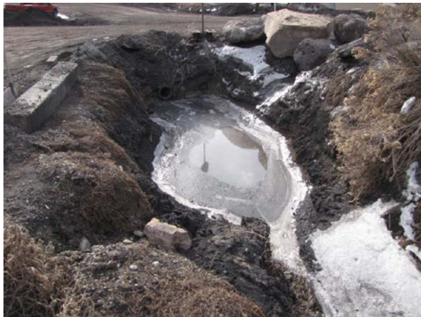
Photo 3 – Sediment Trap East of Bath House
