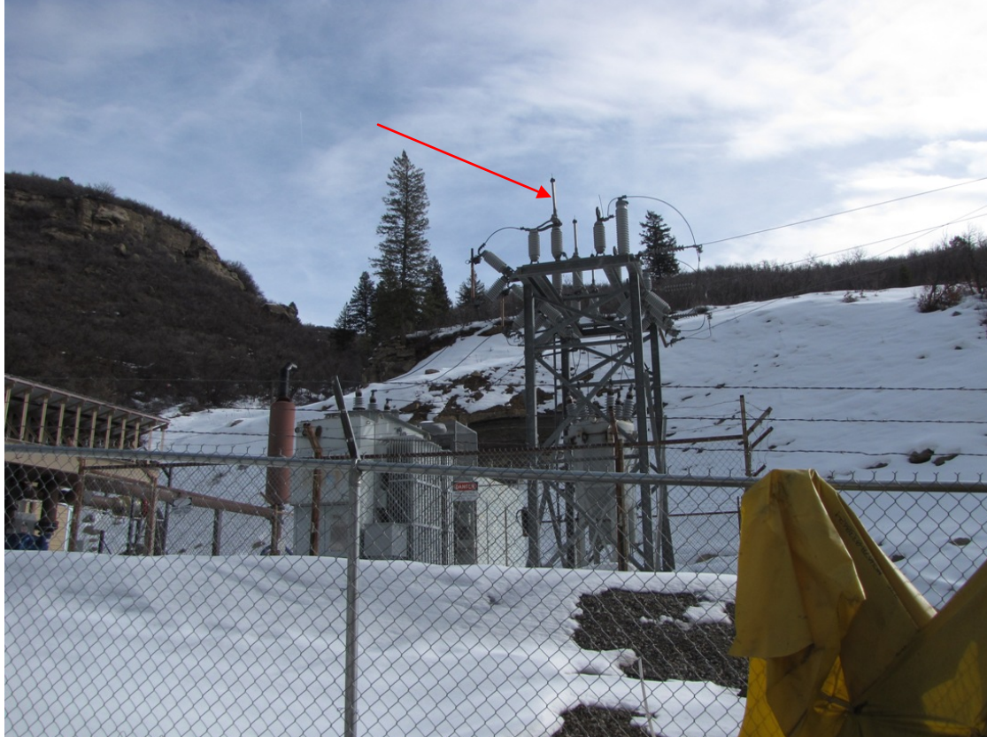
Photo 9 – Open Switches at the Bear Creek Sub-Station
