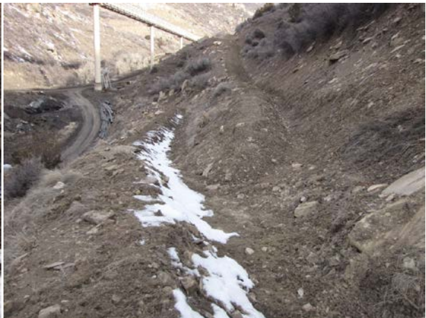
Photo 4 – Clean Water Diversion Above Pond D
