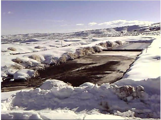
1 st cell of dewater pond system filled with sediment.
