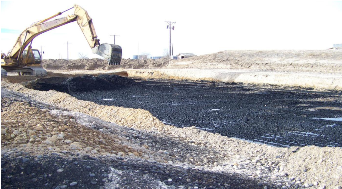
View of Excavation – View Looking Northwest
