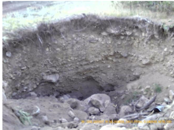
final subsidence hole to fill
