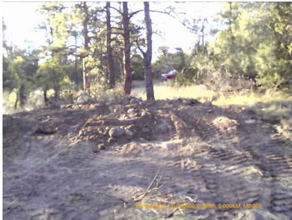
Repairs to subsidence holes
