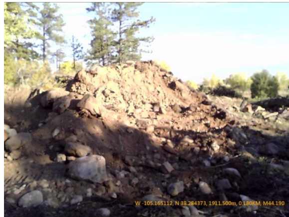
spoil used for fill in subsidence holes
