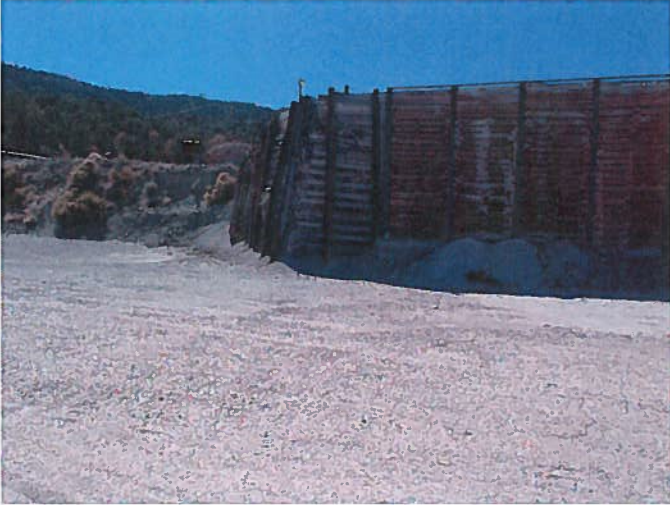
Figure 5: Retention wall constructed on the dump area bench, below the mine area bench.
