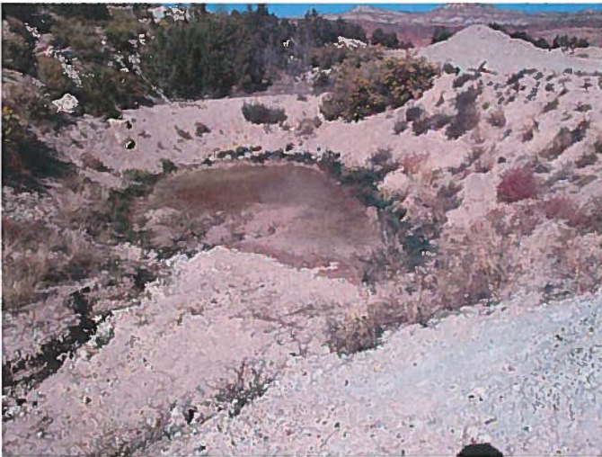
Figure 7: Stormwater retention pond at the base of the dump area bench.
