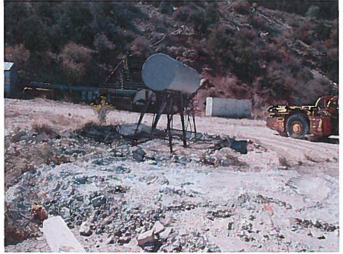
Figure 2: Fuel storage on site. Tank was empty during inspection. Containment will need be enlarged should fuel tank be used in future.
