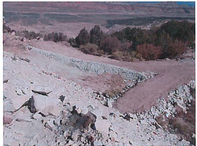
Figure 4: Stormwater retention pond constructed on northwest side of mine bench.
