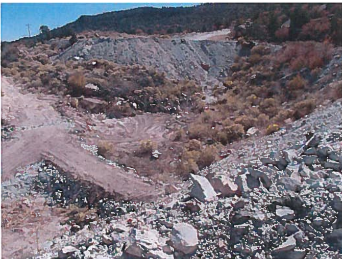
Figure 3: Stormwater retention pond constructed on northeast side of mine bench.
