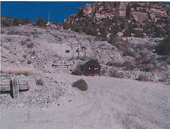
Figure 3: Collapsed JD-9 portal.
