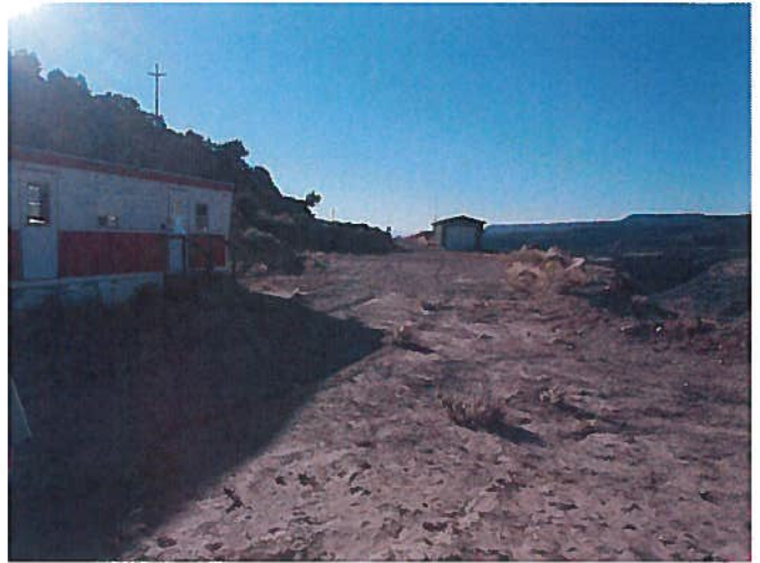
Figure 2: Operation area located above the Wright Portal. Office building in the foreground, compressor building in the distance.
