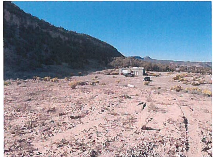
Figure 8: View from reclaimed waste pile area on the north side of Spring Creek Mesa, toward the existing mine building.
