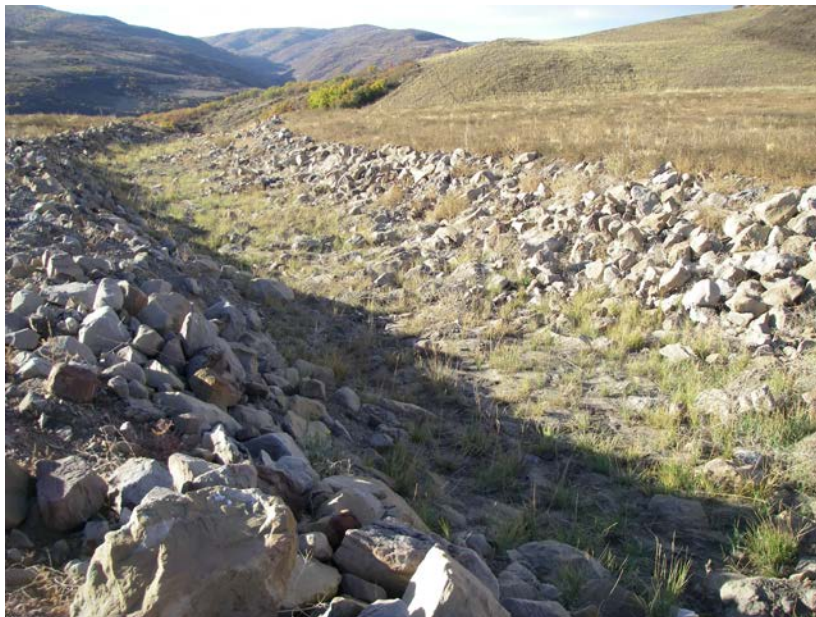
NTEP Ditch – area where additional rock may be needed (pending review of SEDCAD)
