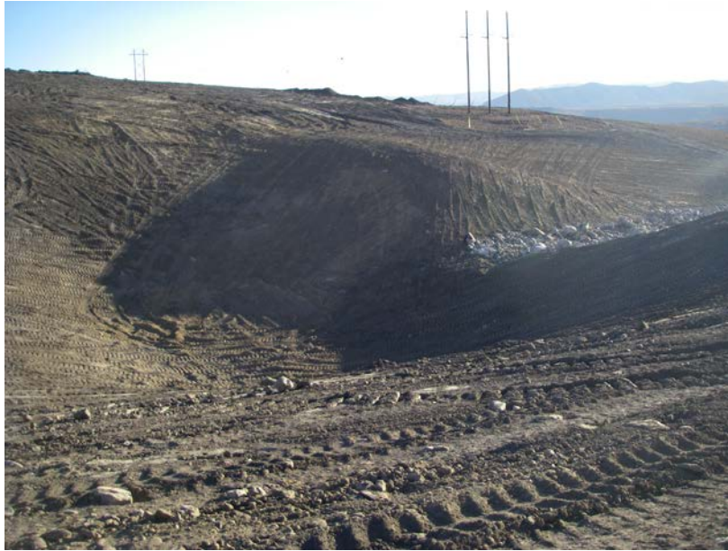
EP2 Pond – after excavation and before final rock placement
