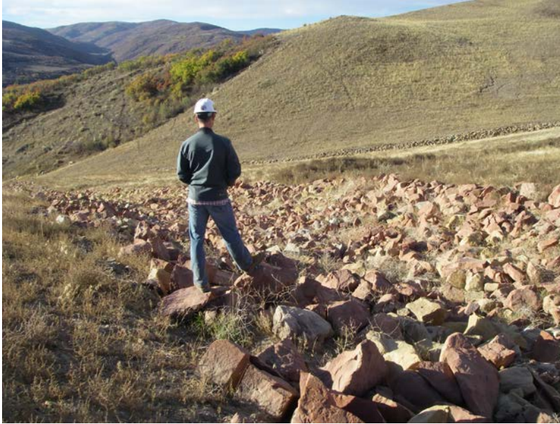
NTEP Ditch – area where riprap coverage is good (below previous photo)
