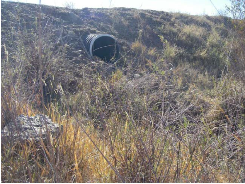
West Ridge Pond – new pipe in primary spillway (corrugated plastic, 42” dia)
