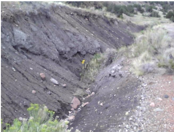
Photo 3: Cut bank that appears to be contributing Additional sediment along west side of FCR92
