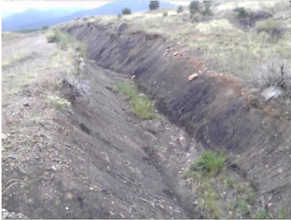
Photo 1: road ditch on W side of FCR92 Note sediment in bottom.
