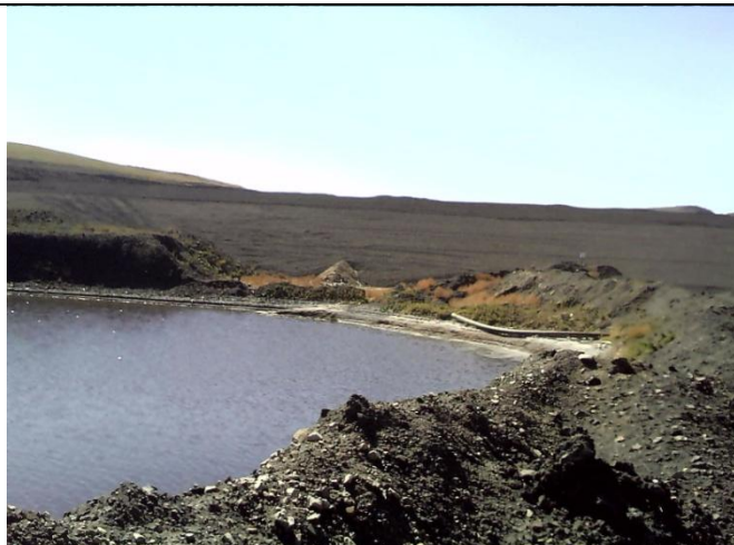
RDA Lift 1 Outslope and Underdrain Outlet
