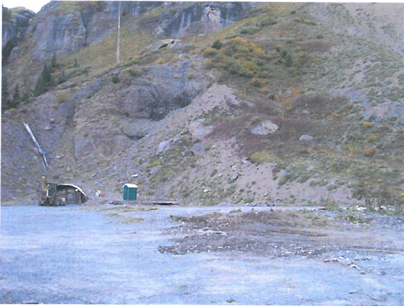
Portal Site - Final Grading
