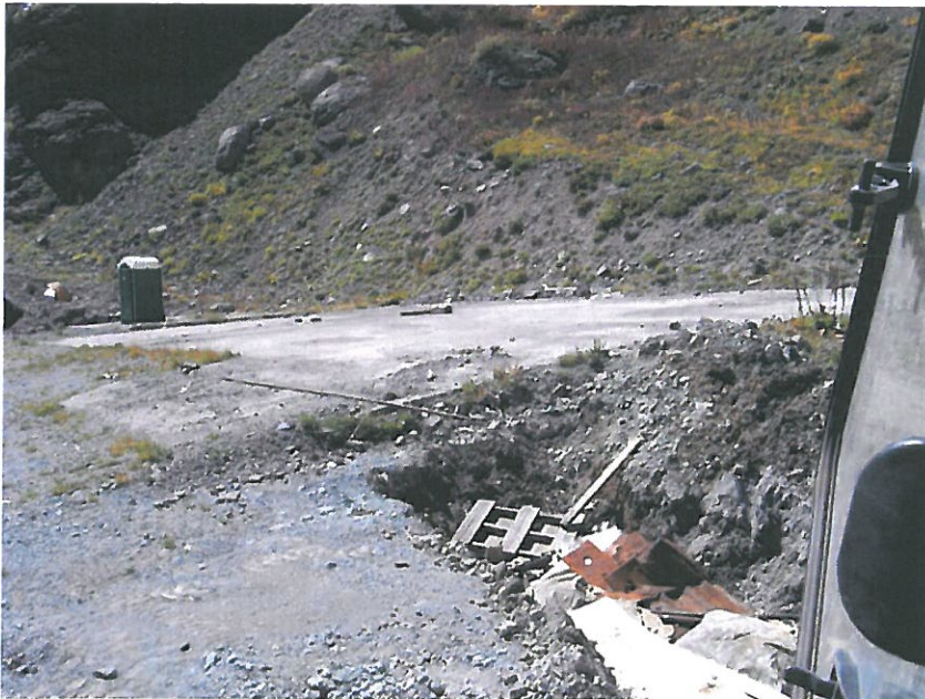
Solid Fill Before final grading
