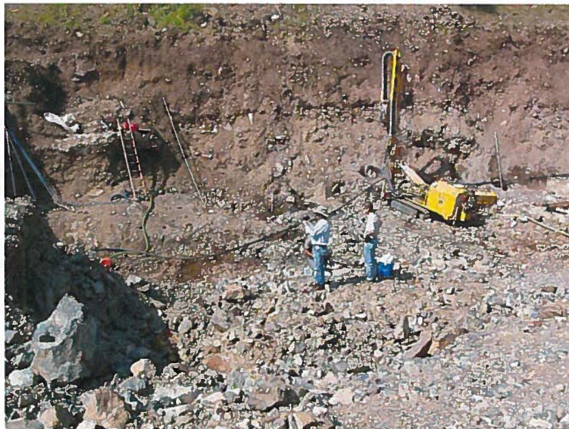
Photo 5 – Inactive drill rig (right side of photo) in grout curtain area that was drilling holes for grout curtain during week prior to this inspection.
