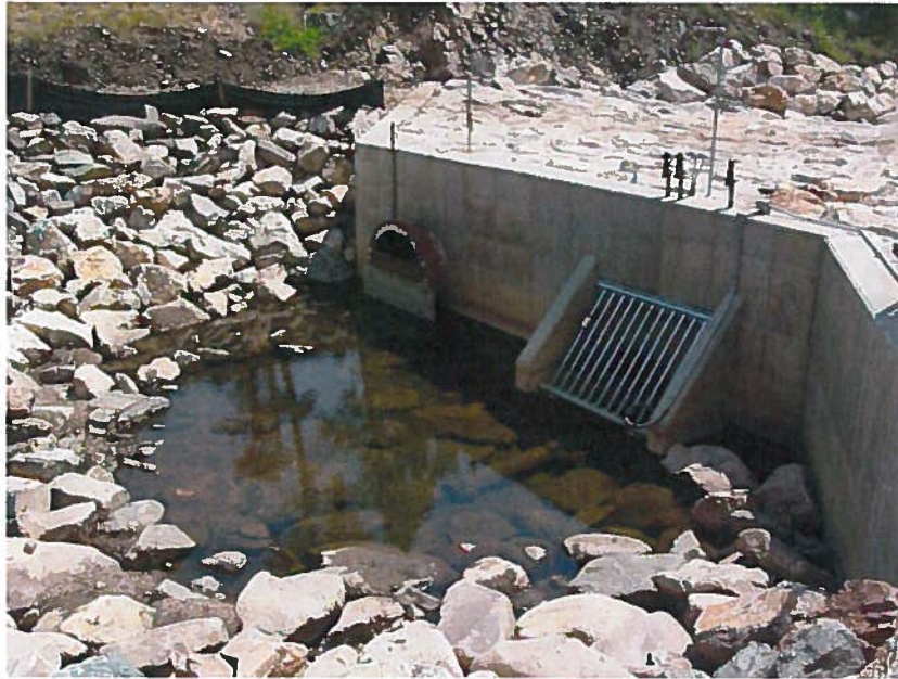
Photo 4 – Ponded Ralston Creek water on upstream side of upper cut-off wall for creek diversion pipeline. 18-inch diameter diversion pipeline is out of view behind trash rack on right side of photo. Steel pipe on left side of photo is stream overflow pipe.
